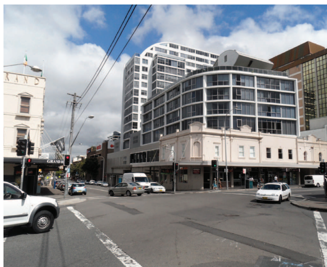
Picture 5.7 Historic Building (Bronte Road/Ebley Street)
