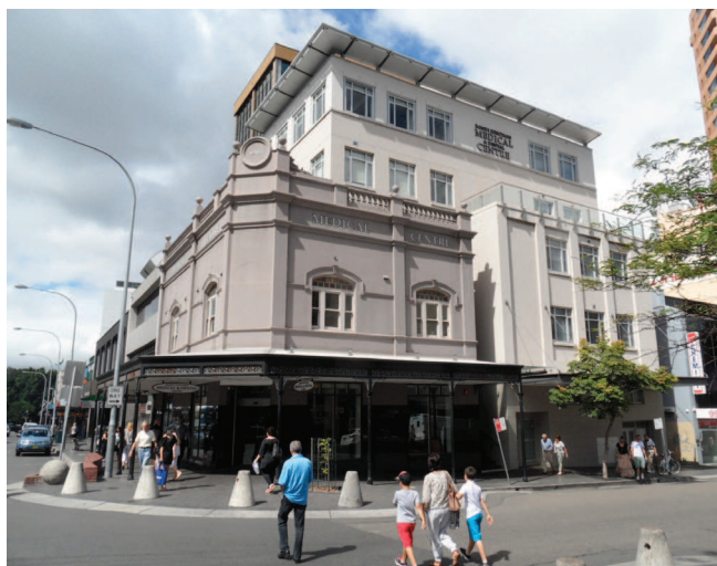
Picture 5.6 Historic Building (Bronte Road/Spring Street)
